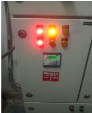
Figure 3 Electrical Measurement by Power Analyzer at Grid Incomer Main Panel
